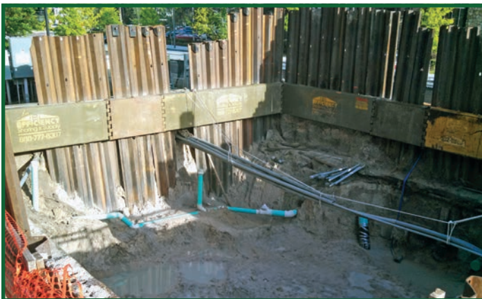
Perfect for shoring around cross-trench utilities
