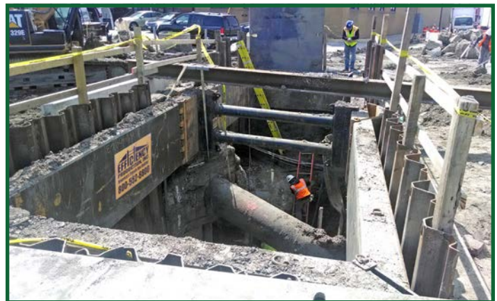
Perfect for shoring around existing structures
