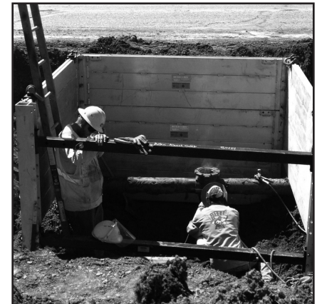
Three-sided configuration with spreaders on long side and removed bottom panels to straddle pipe
