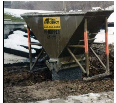
Hi-Hopper in Use
